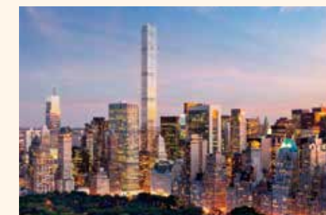
図12 432 Park Avenue 取引価格約95億円 出典/https://ny.curbed.com/building/129/432-park-avenue
